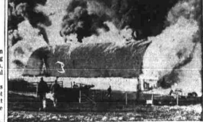
When the barn above was totally destroyed by fire last year, the direct dollar loss to this Midwestern farm family was estimated to be $60,000. Total direct cost of fires to American farmers last year was estimated by the United States Department of Agriculture to be more than $150,000,000. The USDA and the National Fire Protection Association are co-sponsors of Fire Prevention Week, Oct. 7-13.
