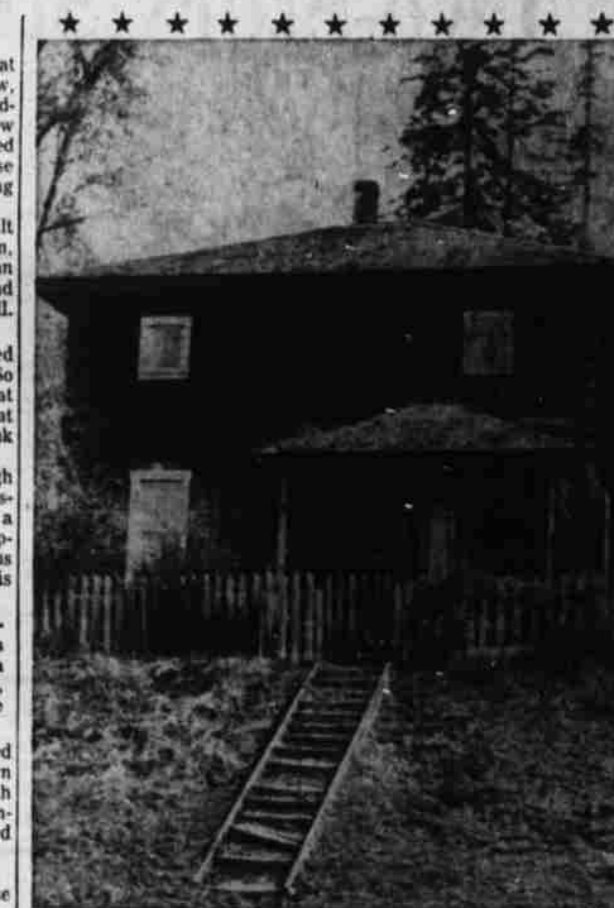
MEHAMA—This hand-hewed log house at Freres' old mill, above Me-hama on the House Mt. Road, was built nearly 70 years ago by Billy Smith. His only help was a horse. (Statesman Photo).
