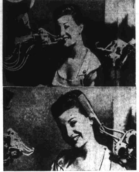
CHENECTADY, N. Y .-- Model Ruth Feldheim gets a beauty treatment, lipstick, hair-do, and all from the "Yes-Man," the two-armed electro-hydraulic "slave" developed by General Electric engineers here. The dexterous mechanical device, designed primarily for chores in dangerous radioactive areas, duplicates motions performed by an operator with a twin "Yes-Man" from a remote point. (AP Wirephoto)
