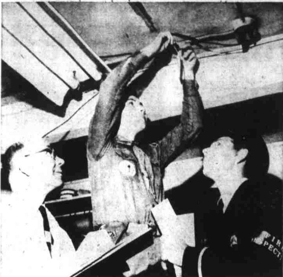
Downtown businesses are getting a fire prevention inspection this week as some 50 agents representing insurance companies plus Salem firemen and boy scouts make a door-to-door check of fire hazards. Inspector Robert Burke, Oregon manager of Deans and Homer, underwriter managers, Portland, is shown above at left watching Salem Boy Scout Ronald Meola tag a faulty electrical cord in a downtown business house. Fireman Clarence Nelson is at right. The safety inspections will conclude today.
