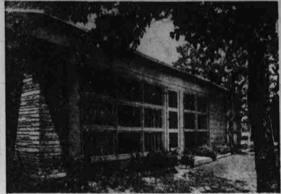
OVERHANGING EAVES to keep the summer sun from heating a house through large window areas have become even more important with the spread of air conditioning. As shown here, floor-to-ceiling window walls can be completely in the shade at midday in summer. When the sun is lower in the sky in winter it can shine in the windows. Such overhangs are carefully planned. They have to be wider in Minneapolis than in Dallas.
