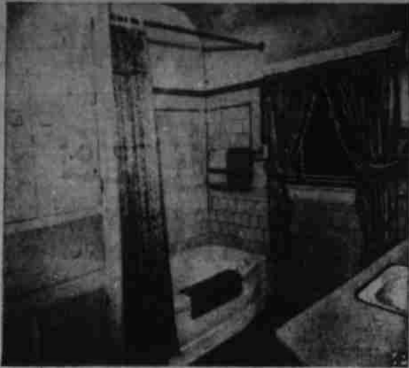
THE SAME BATHROOM after modernization. A new tub is placed away from under the window. Walls have been tiled and an up-to-date vanity lavatory has been installed. Package remodeling, such as this, is arranged by many plumbing contractors carpentry, tile setting and painting.
