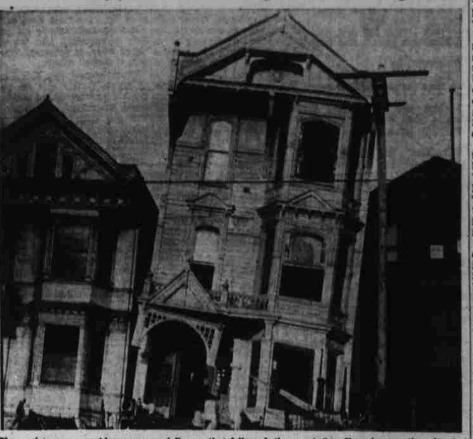
These picturesque residences escaped flames that followed the great San Francisco earthquake, but the one in center was shaken off its foundations by the tremendous earth jolts and had the appearance of the Leaning Tower of Pisa. A resident poses in the doorway while doubtless speculating about the cost of renovations.
