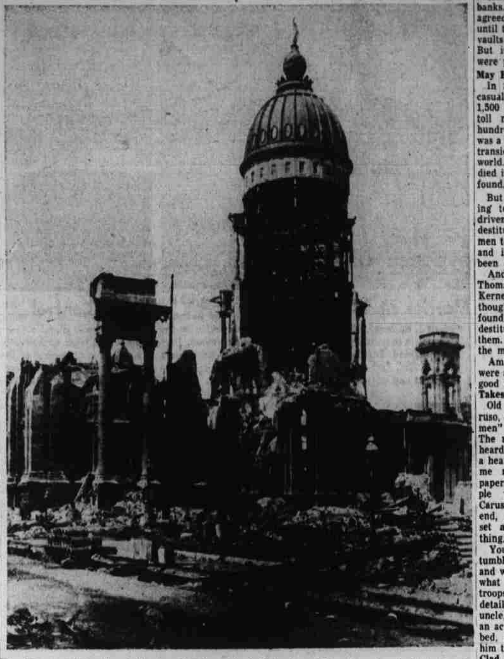
The fire-ravaged cupola of the San Francisco city hall stands starkly against the sky following the catastrophic earthquake and conflagration which struck the Bay City on April 18, 1906. While the cupola refused to collapse, remainder of the structure was reduced to ruin and rubble as were numerous other public buildings in the city. This and other photos on this page were loaned to The Statesman by John Freeborn, 1610 N. Church St., and were taken by a sister, Nelly Freeborn, Osborne, Kansas, who was in San Francisco at the time of the quake.
