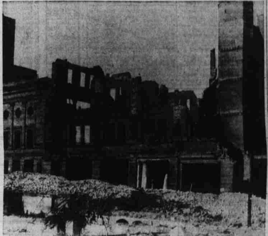
All that remained of San Francisco's YMCA building (above) after the 1906 quake and conflagration was charred, broken walls. Masses of brick shaken loose by the earth jolts can be seen piled in front of the structure. Few were the business and public buildings which escaped damage in the catastrophe and death toll was placed at 452 persons. Damage ran to $350 million.
