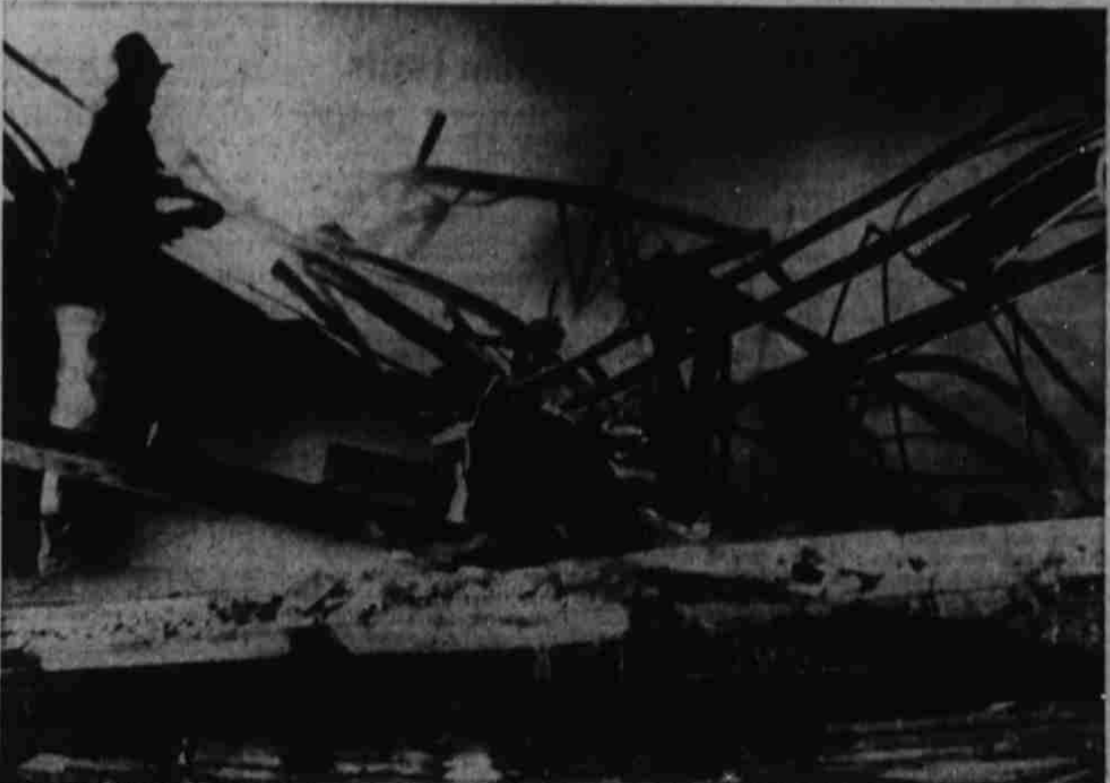
INDEPENDENCE—Nothing was left of the Holt Equipment Co. machine shop Saturday night except twisted steel and debris as a fire with an estimated damage of between $500,000 and $1,500,000 swept through that portion of the plant. One of the firemen from the three companies in attendance (Monmouth, Dallas and Independence) checks a stream of water on the smoldering fire. The firm plans to rebuild the plant. (Statesman Photo by John Erickson.)
