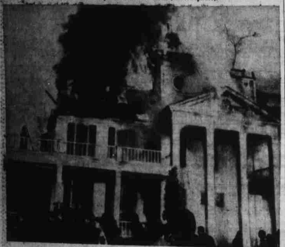
School Burns SALTSBURG, Pa.—Firemen standing on porch roof aim futile hose lines on flaming upper portion of Kiski Prep School central building during fire Thursday which ruined frame structures. School president estimated damage at $300,000 to $500,000. Twenty-three students and faculty members fled burning building uninjured. (AP Wirephoto).
