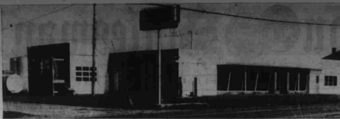
"Open for business" will be the sign on this new Oregon State Farmers Union building at 3615 Silverton Rd. Wednesday morning. The official opening, to which both Farmers Union and the general public are invited, has been set for Feb. 13. State Farmers Union officers will inspect the building next week when the annual Oregon State Farmers Union convention gets underway here. (Statesman Photo)
