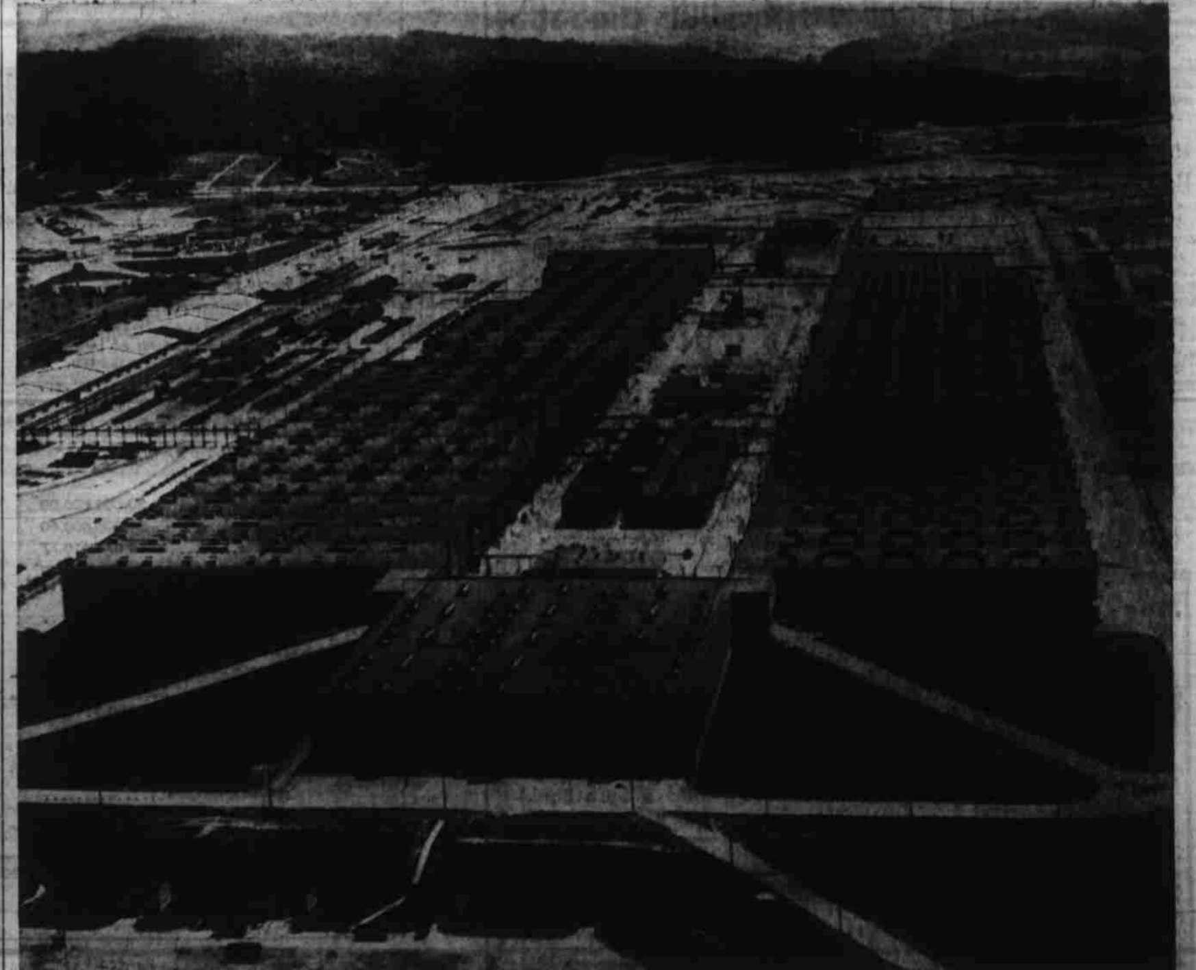
NASHVILLE—The Oak Ridge Uranium-235 production plant is the largest continuous and four stories high. Above is a view of the "K-25" gaseous diffusion plant—gaseous process-plant in the world. Each side of the giant "U" is half a mile long for the separation of fissionable uranium-235 from normal uranium.
