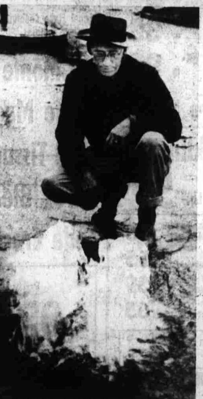
Artesian Well? Elmer Harris, city streets employee, is shown looking at what appears to be an artesian well in the middle of E. Miller Street Wednesday afternoon. It occurred when the street's storm sewer backed up forcing water out this manhole. (Statesman Photo).
