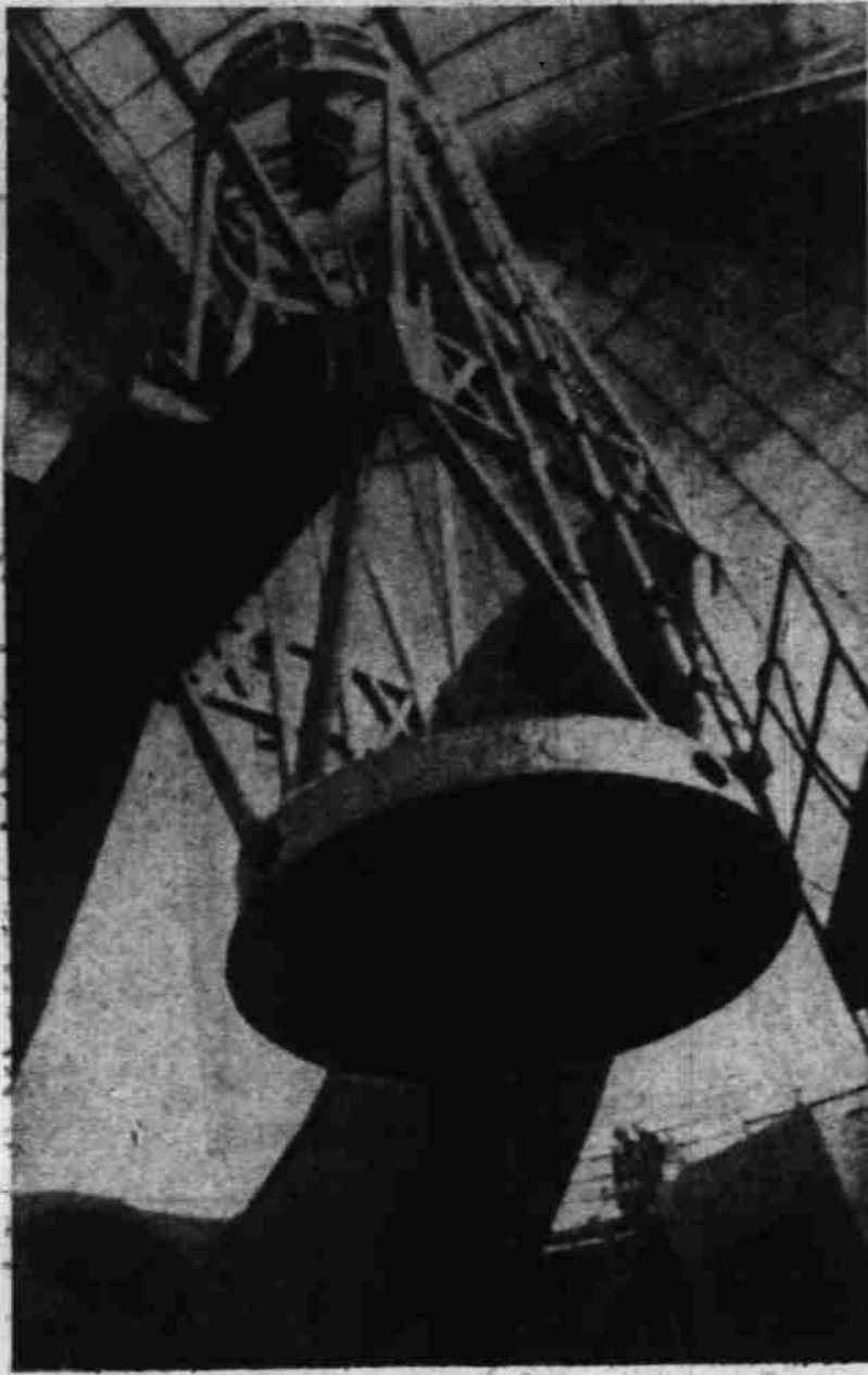
To Watch Sky MT. HAMILTON, Calif.—Huge frame of new 120-inch reflecting telescope at Lick Observatory stands ready for ten-foot mirror disc that will make it an operative instrument—second largest telescope in the world. Huge metal arms support telescope frame, the whole so delicately balanced that it is easily turned by a 1/25th horsepower motor. (AP Wirephoto).
