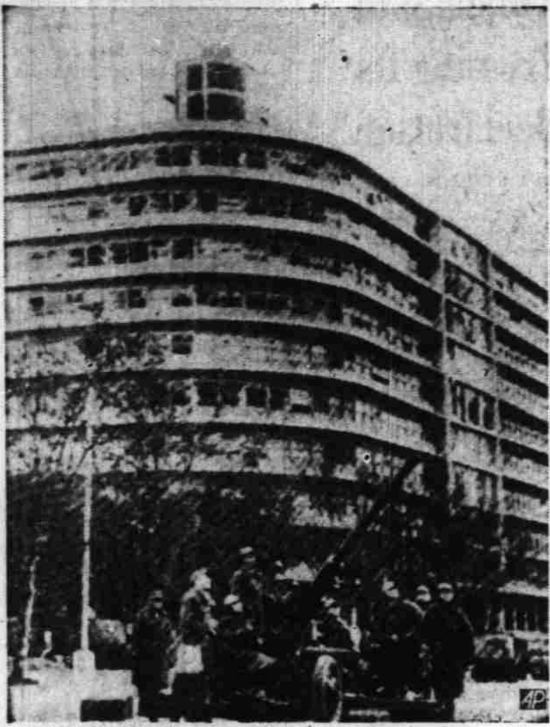
BUENOS AIRES—The Navy Ministry building in Buenos Aires, stronghold of rebels during the bloody fighting in Argentine's capital, is shown after its surrender. Almost all windows are broken. In the foreground is one of the anti-aircraft guns used in the fighting. The Army has taken complete control of Argentina. (AP Wirephoto via radio from Buenos Aires).
