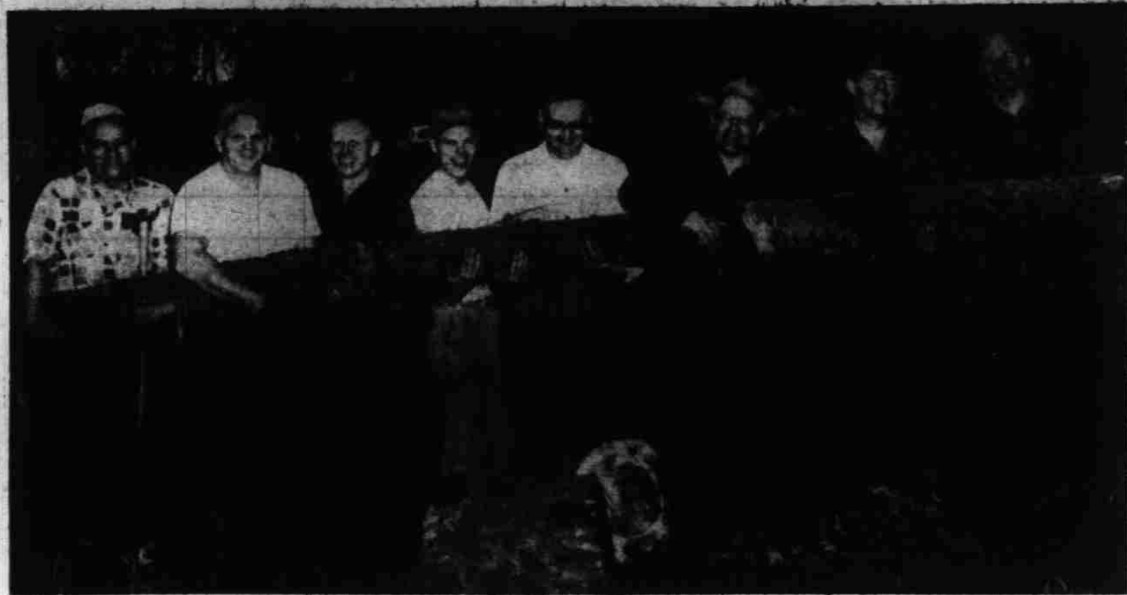
Members of the Salem Kiwanis Club Wednesday took their turn at clearing Wallace Park preparatory to its being put to use for picnic purposes this summer. Tuesday, Junior Chamber of Commerce members launched the two-week clearing program; today Isaac Walton League members take over. On left is Park Supt. Walter Wirth. Fourth from left is Raymond Gotchall, Jaycee member in general charge of the program. The others, from the left, are Kiwanis members Obe Wiltis, Phil Brownell, William Gaarenstroom, William Hammond, William Johnston and Salem's Mayor Robert White.
