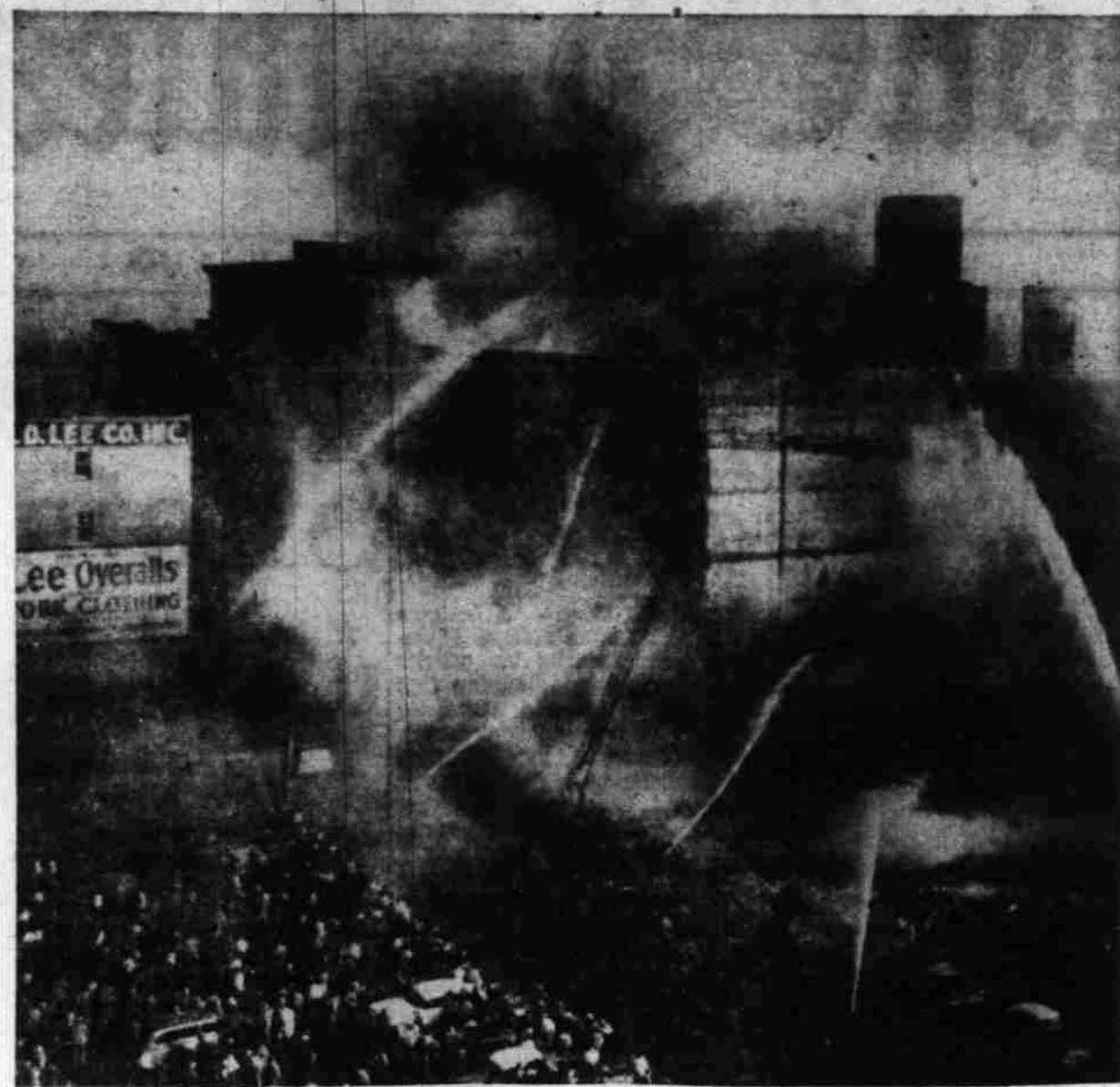
MINNEAPOLIS—Firemen feed water onto the six-story W. S. Nott building here after flames had already destroyed the Nott annex, lower right. The firm manufactures fire protection equipment. The blaze late Friday apparently started in the annex and then spread to four other industrial buildings, including the eight-story Fur-Tex building, across a street to the left of the Nott main building. (AP Wirephoto)
