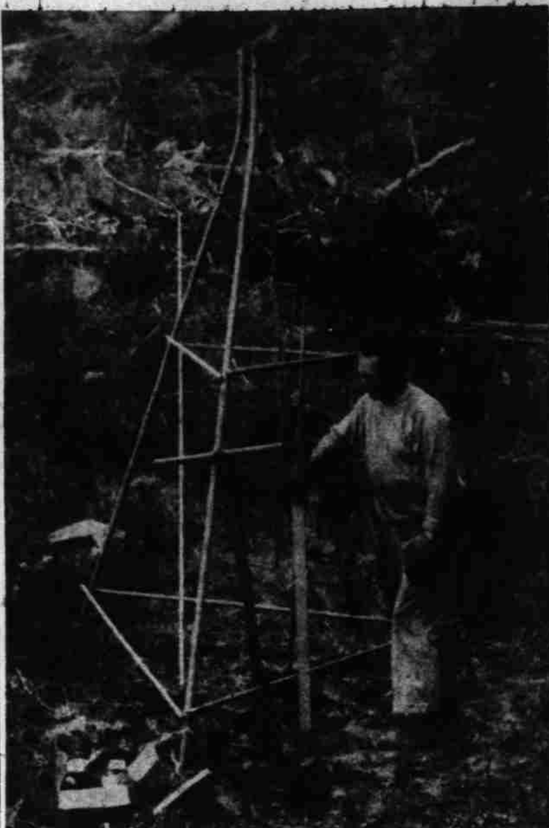
SILVERTON—Erecting home-built drilling rig on his mining claim in Wilhoit Springs area, 14 miles northeast of Silverton is Lester Johnson, 5169 Verda Lane, Salem. Johnson began drilling Saturday for uranium or other radioactive substance that could spell big money. (Statesman Photos)
