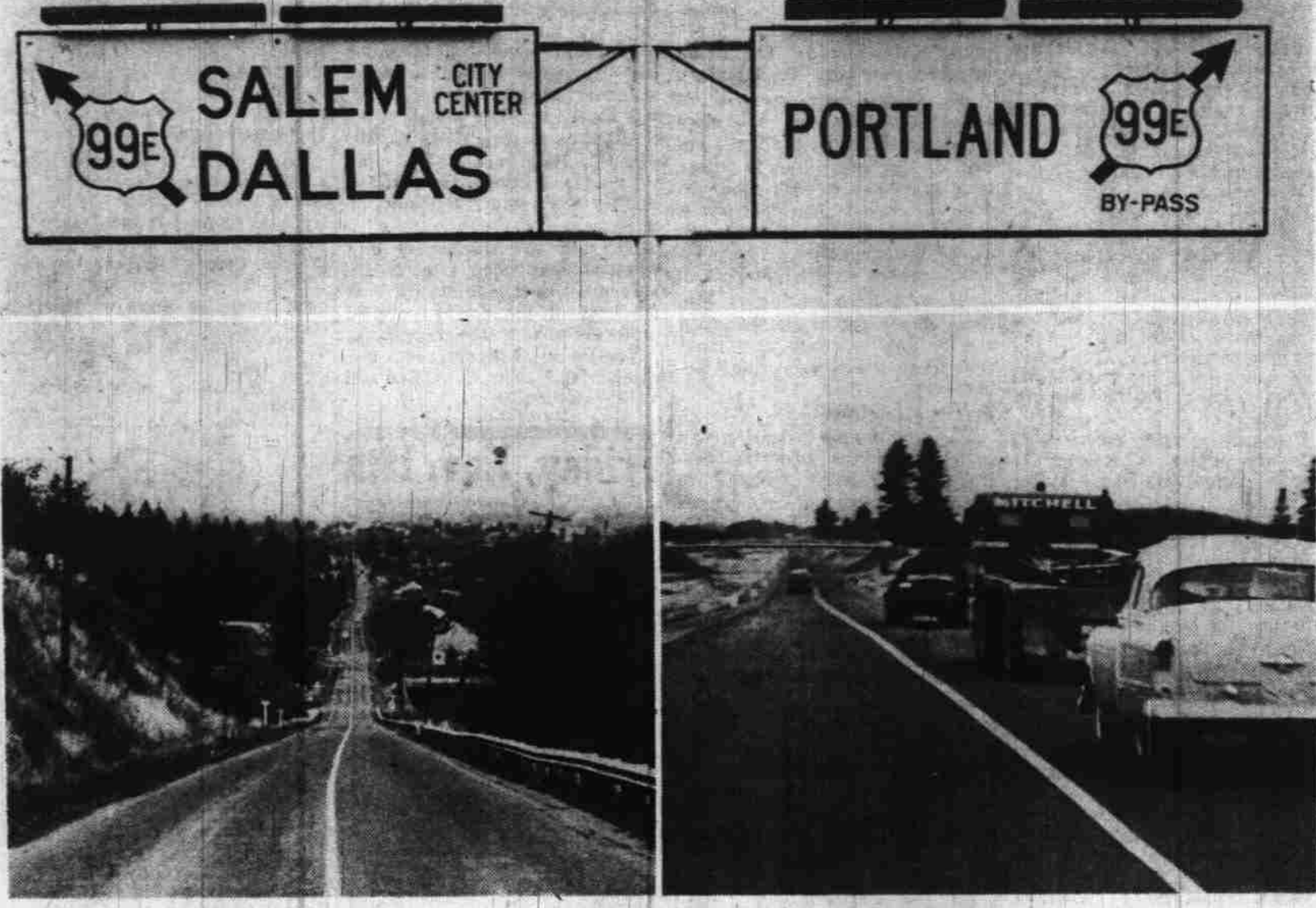
Subject of bitter complaint by many tourist catering businesses, the Salem by-pass is shown above along with its effect on 12th Street traffic. Top photo shows sign which has been criticized by affected businessmen as leaving the impression that the by-pass is the principal route and that route to the left is merely the way to Dallas via Salem. Bottom left photo shows deserted 12th street while photo at bottom right shows traffic on by-pass route. (Statesman Photo)
