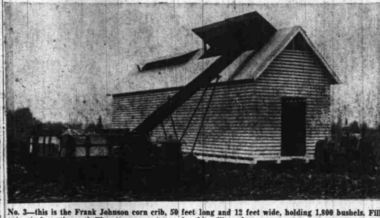
No. 3 —this is the Frank Johnson corn crib, 50 feet long and 12 feet wide, holding 1,800 bushels. Filling is from the roof. There's no scooping or hand-handling of corn necessary.
