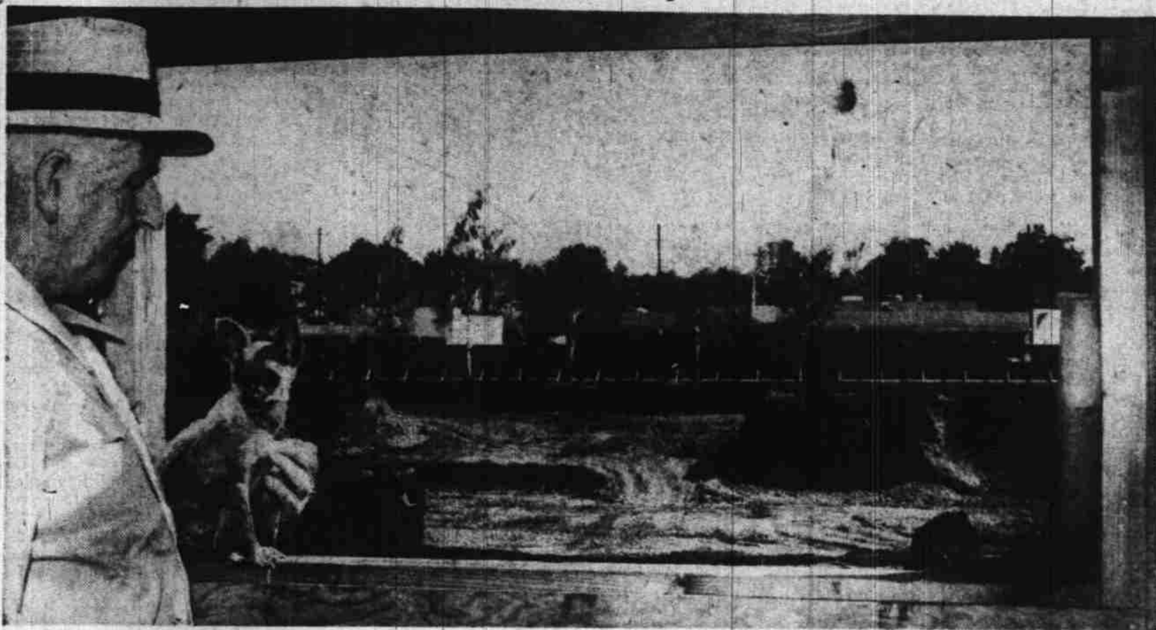
On hand for the start of work on the new Meier & Frank Department Store building, M. V. McKee, 643 Union St. and his Chihuahua dog 'Subie' are shown at one of the 'sidewalk superintendents' windows which surround the excavation waiting for work to begin. Not much happened, though. Workmen said it would be the end of the week before viewing would be worthwhile. McKee thought his tiny dog was impressed with the size of the diggings, however. (Statesman Photo.)
