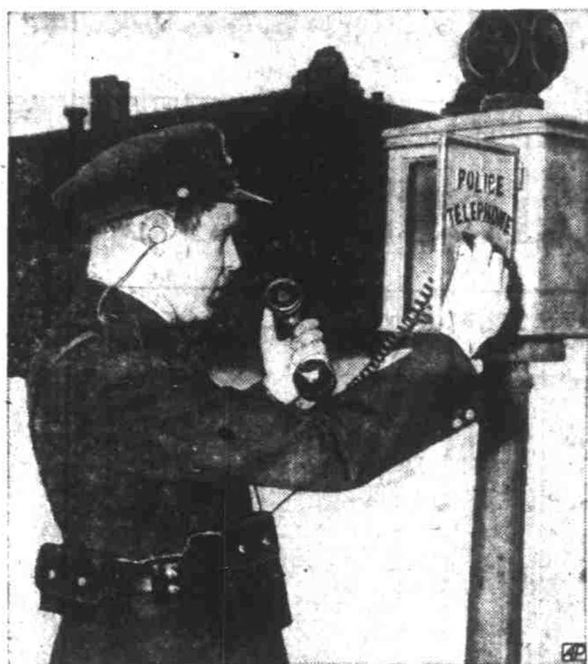
ST. LOUIS—Patrolman Joseph Elke of the St. Louis police force wears the new two-way radio designed for foot policemen, but uses the old telephone call box.
