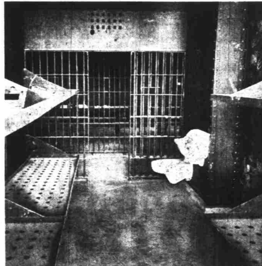
Heavy steel walls and doors characterize the detention department atop the building. Shown above is a typical jail cell in the adult division. Shelf-like items on the sides are all-steel bunks. There are separate sections for men, women and juveniles.
