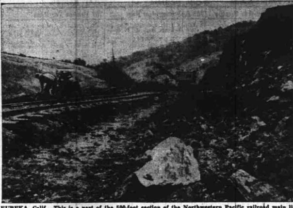
EUREKA, Calif,-This is a part of the 500-foot section of the Northwestern Pacific railroad main line near Eureka, Calif., that has to be straightened as much as 40-inches a day because a moving hill, right, keeps pushing it towards Eel River, left of the tracks. The hill has been giving the railroad trouble since the line was built in 1916. Recent heavy rains are the cause of the current "push." In 1938 the hill really got out of hand and the line was tied up for 73 days. (AP Wirephoto to The
