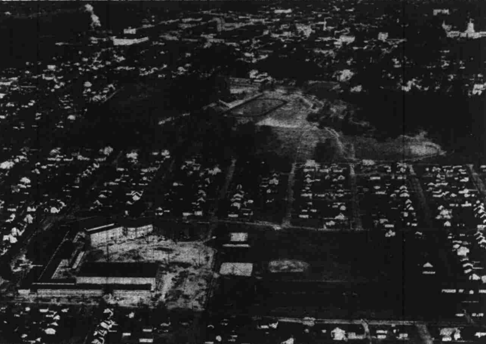
This aerial photo was taken over South Salem, looking northwest, and shows the extent of the new South Salem High School and Leslie Junior High in foreground. Center is Bush's Pasture, with the Willamette football stadium and track, and at the upper left is the Willamette River and bridges. Upper right is the statehouse, with Salem's business section at upper center. Photo is No. 2 of a series taken specifically for The Statesman by this newspaper's photographer, John Ericksen.
