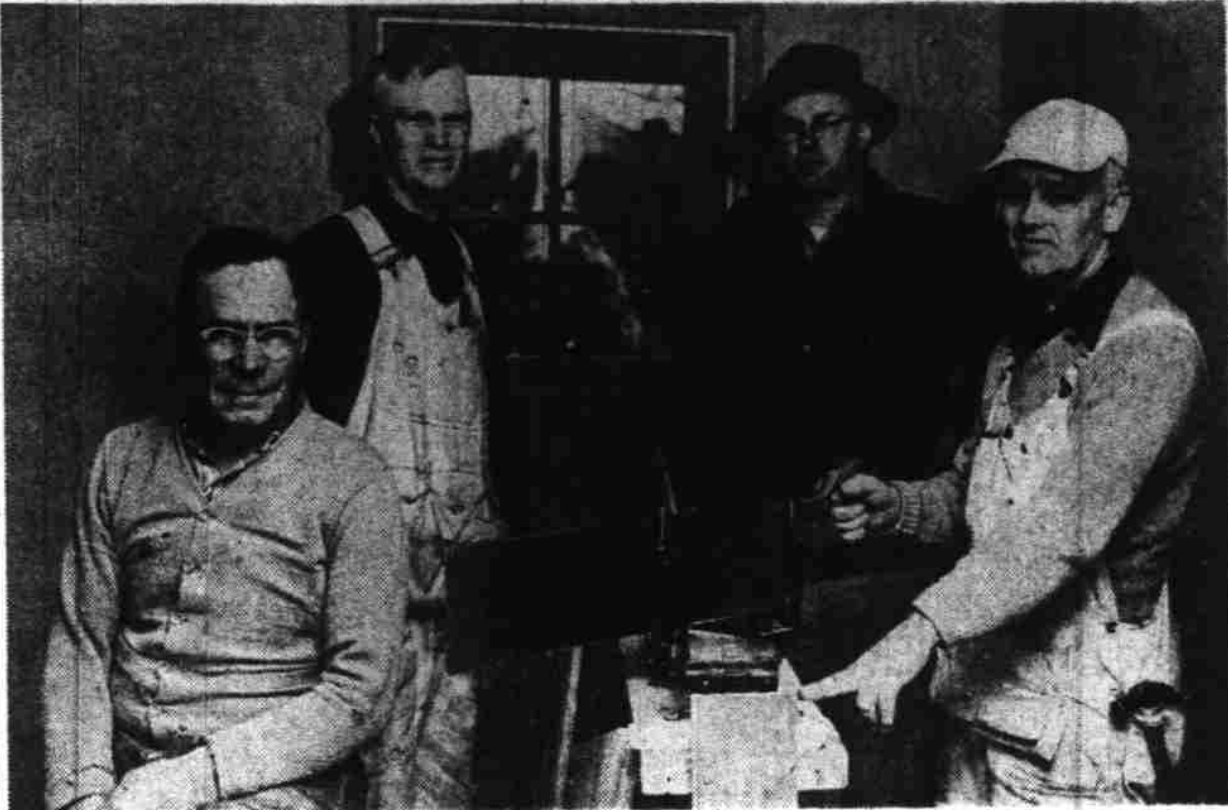
SILVERTON—A Sunday School and Youth addition to Trinity Lutheran Church at Silverton which was estimated at $25,000 will come to about $15,000 because of donated labor. The report was made at annual meeting of the congregation Wednesday night. Among those putting in a lot of free-time are from left to right, Silas Trovond, chairman of the building committee; Jelmer Refsland, in charge of construction; Harlan Moe, president of the congregation and Martin Hatteberg, assistant to Refsland. (Statesman Farm Photo.)
