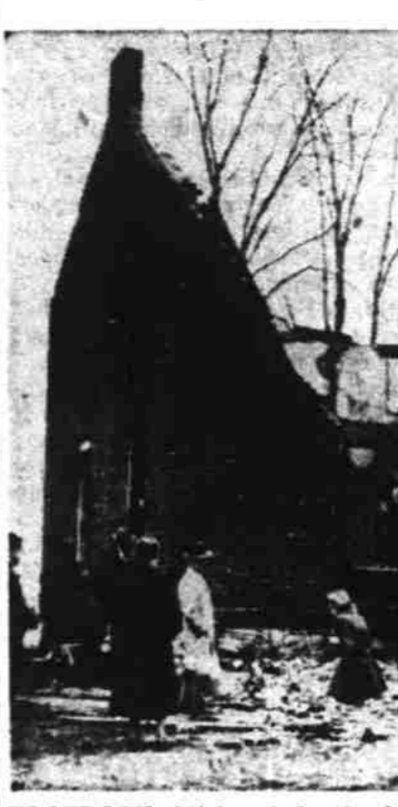
FLATROCK, Mich.—Only the brick walls stand where Mrs. Mary Hurst, 25, and her four small children perished in the flames of their home in Flatrock, Mich., on Christmas day. Townspeople inspect the gutted home. (AP Wirephoto to The Statesman)
