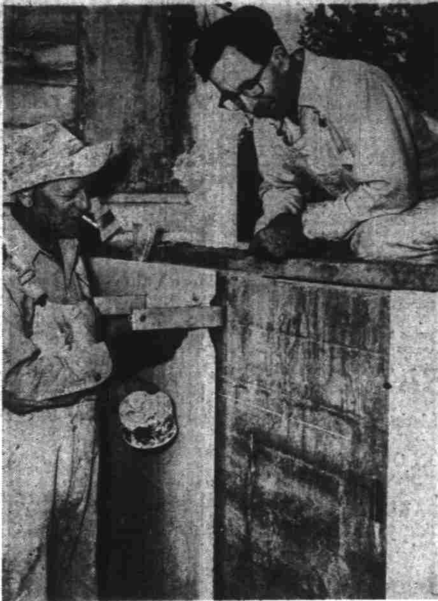
Engrossed in the skill-demanding job of fixing a slab of exterior marble facing to the new Marion County Courthouse building in Salem these two marble "mechanics" carefully measure a section. Ed Linder of Los Angeles, Calif., (left) works on a slab while Lloyd Allan, Portland, foreman of the Lutz Marble Co. crew, looks on. Allan has been a marble "mechanic" for 25 years.
