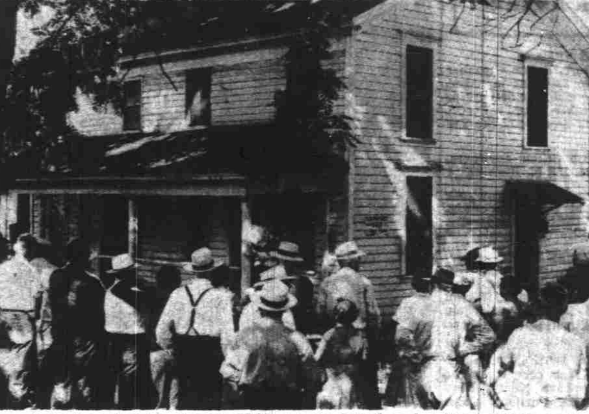
Low point in the life of this 112-year-old house came Saturday when it was sold by Auctioneer Claude Kilgore (on porch) to wreckers for $35 to make room for the new school administration building at 13th and Ferry Streets. But this, Salem's second oldest house—originally a pioneer Methodist parsonage—may yet be saved as a museum if efforts of the Marion County Historical Society to raise funds for moving and restoration succeed. (Statesman photo.)
