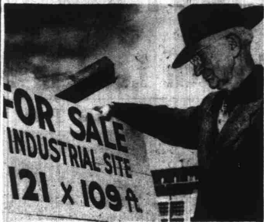
A. M. Hansen, Salem pioneer business man, inspects real estate sign at the leveled-off site where Hansen's old, historical wood-working mill stood for 50 years at Mill and South Church Streets. The mill, oldest of its kind in Salem, was torn down recently.
