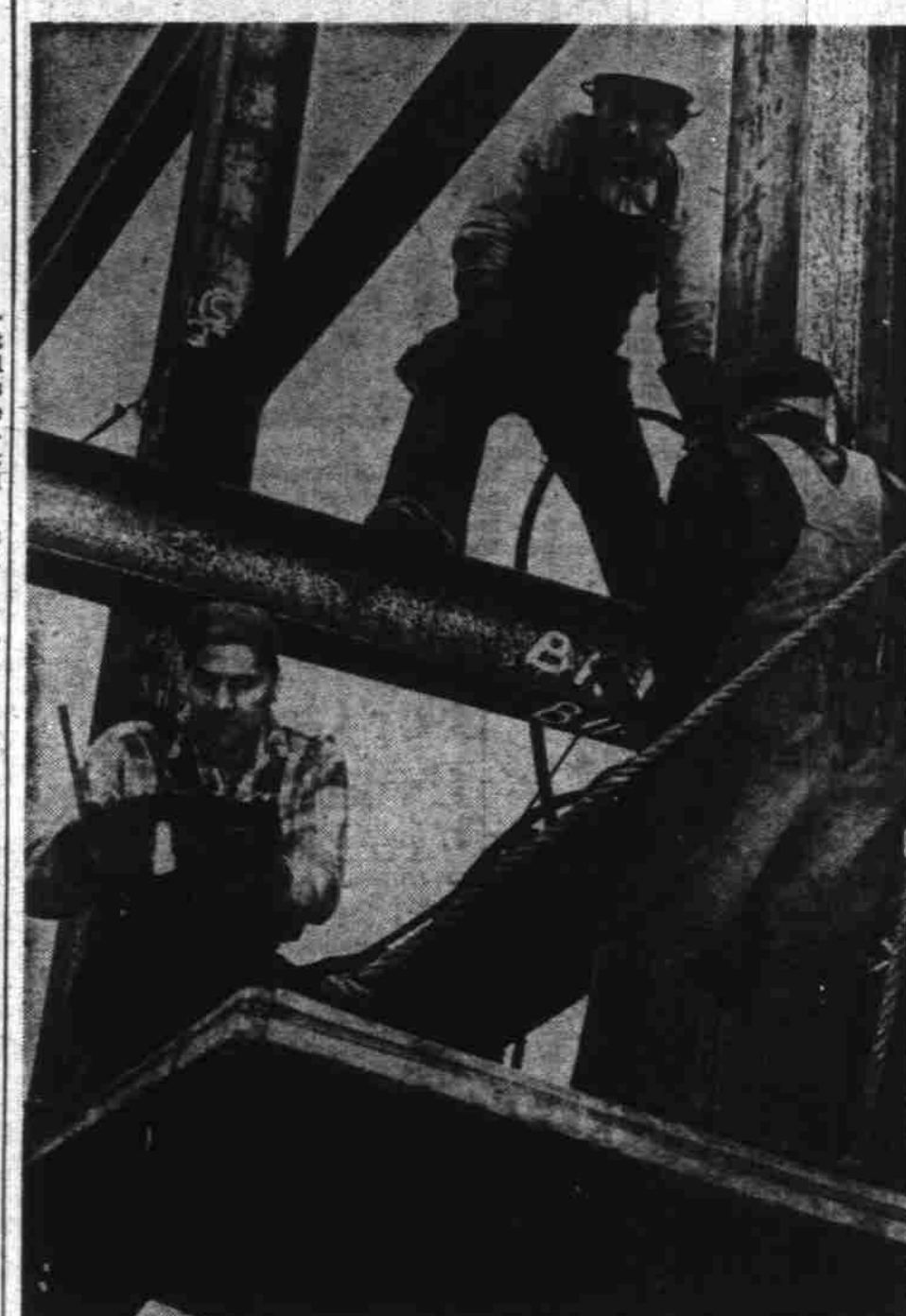
It's noisy business as these three Portland iron workers start riveting on the steel skeleton of the new Marion County Courthouse. The men (from left), Art O'Burn, Bill Adams and T. Tye, are on the ground floor this week, and plan to be working on the second story by Tuesday. The white streak on the left is a red hot rivet. (Statesman Photo.)
