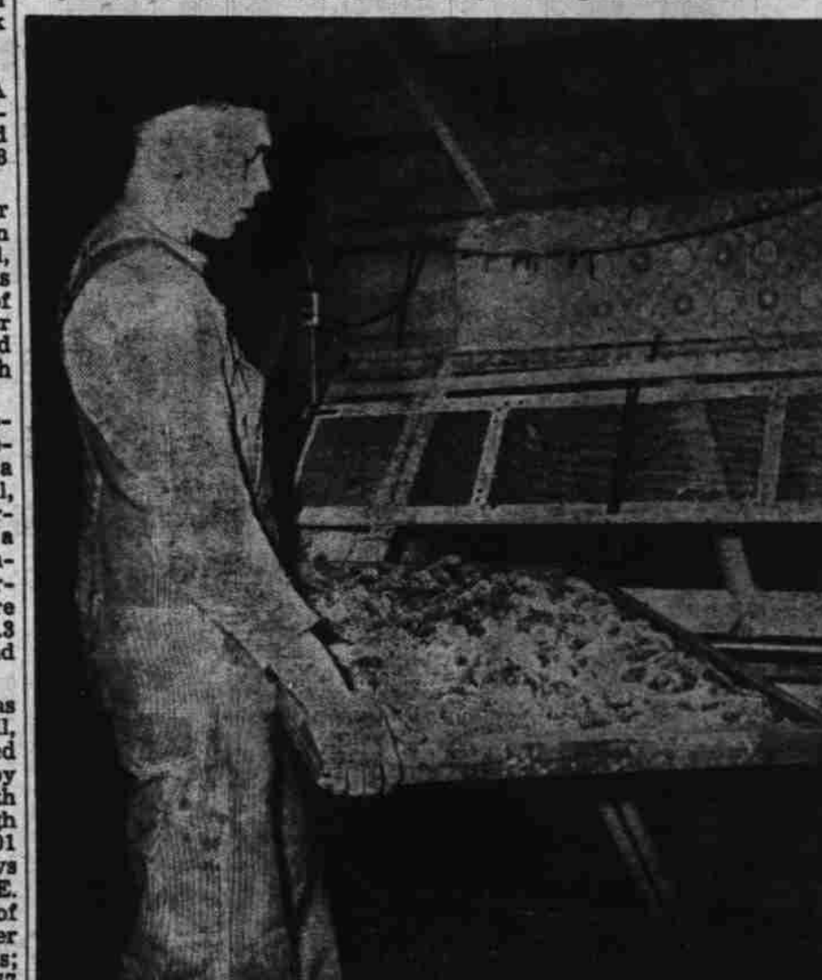
An employee of the Woods Tree Seed Company puts a tray of cones into the drier—a converted prune drier. The cones are cured at slow, steady heat. (Photos by Homer Lyons, Oregon State Board of Forestry.)
