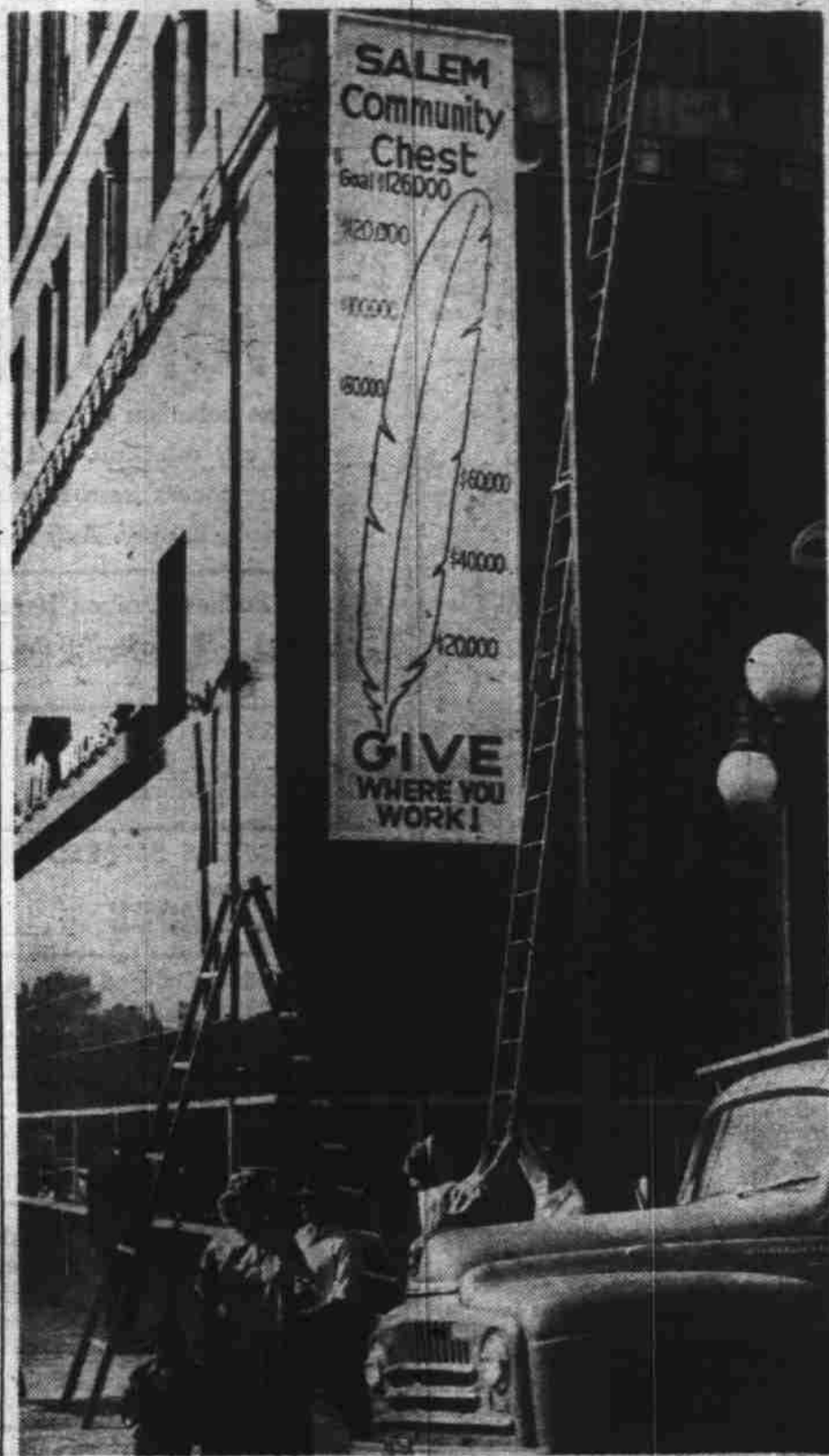
New "tenant" at the downtown Livesley Building is a 20-foot Community Chest sign on which fund drive progress will be charted up the red feather symbol toward the $128,000 goal. General solicitation in behalf of 20 youth and welfare agencies started Wednesday. All materials and work on sign was volunteered. (Statesman Photo.)
