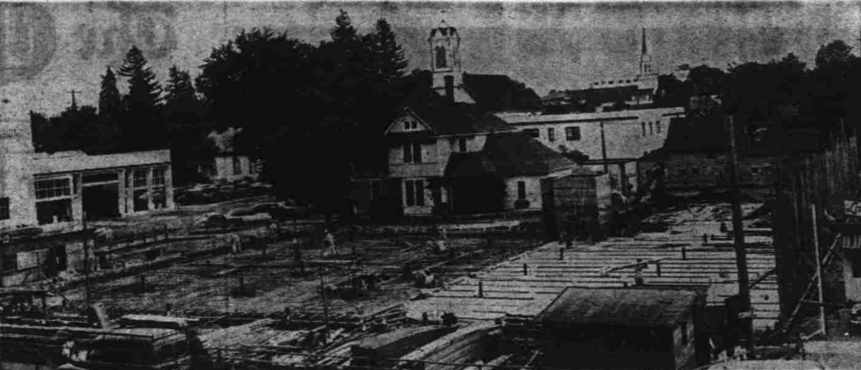
Construction of The Oregon Statesman's new $300,000 building at North Church and Chemeketa Streets neared the half-way point this week with the pouring of the 9 1/4-inch concrete first floor. Photo shows the south end already poured, with reinforcing steel
