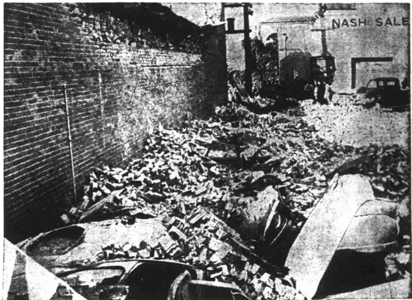
FRESNO—Thirty automobiles and trucks were covered when the building of a Fresno, Calif., garage collapsed. Fire department officials called to the scene attributed the destruction to heat expansion. The building had just been reroofed. No one was injured or killed, though only seconds before the crash, a man had parked a car next to the building. (AP Wirephoto to The Statesman.)
