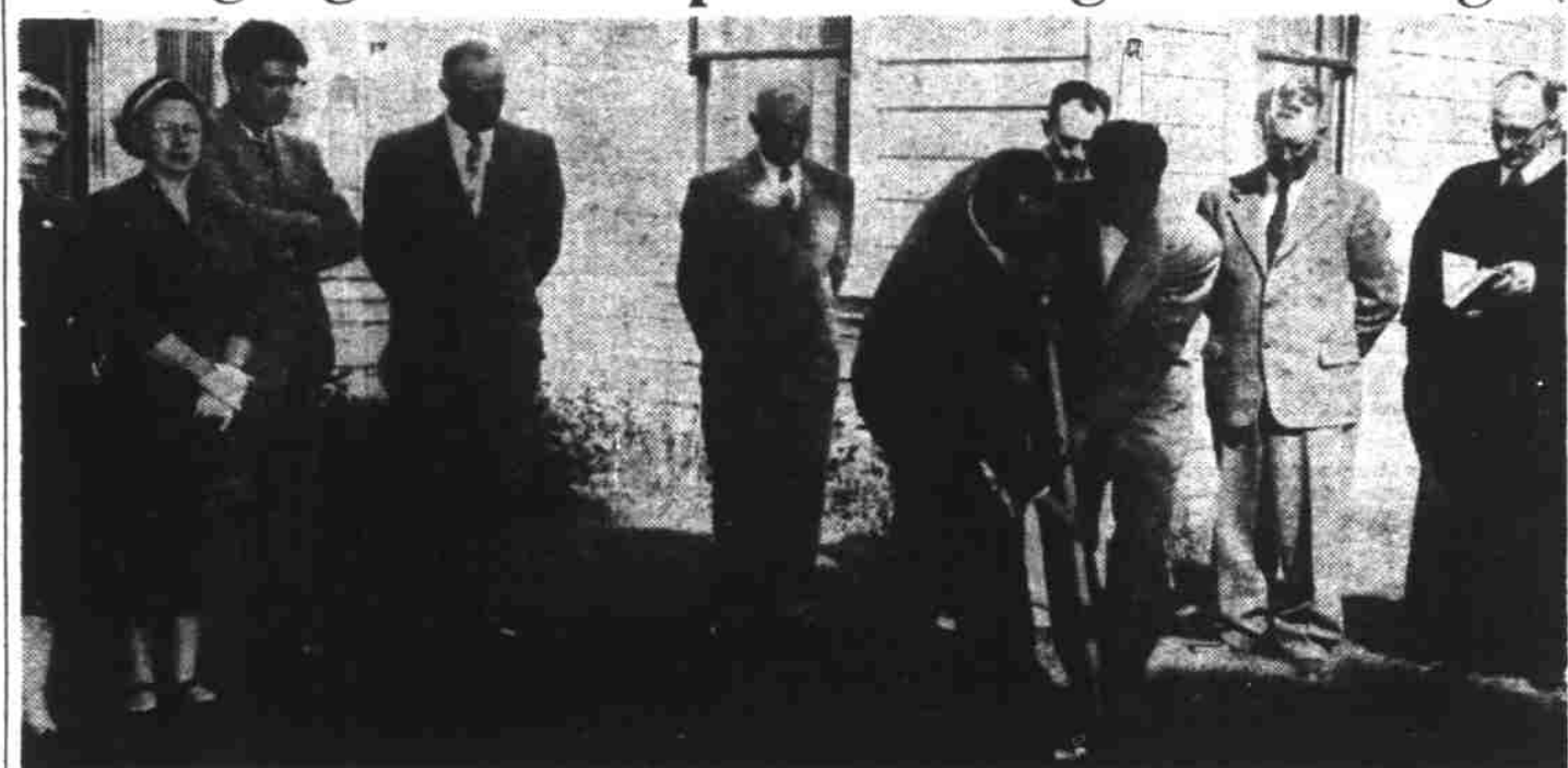
SILVERTON—Ground has been cleared this week for construction of the new Methodist Church at Silverton. In foreground, building committee chairman, Ben Sprick, pastor, the Rev. Douglas Harrell, is at the right, while in the background are other members of the building committee including Mrs. Floyd Fox, Mrs. W. Dale LaMar, Dr. Norman E. Dodds, E. A. Finlay, Edgar Boyce, James L. Payne, the architect, and Harry L. Riches, treasurer.
