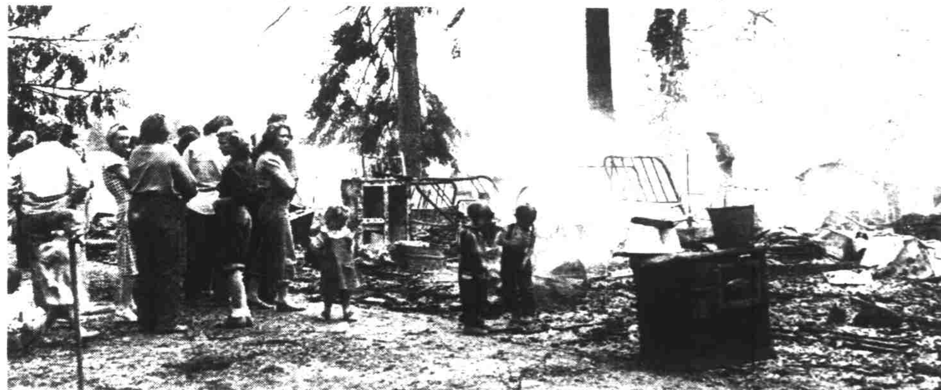
Hoypard workers, many of whom lost all they owned, survey the smoldering ashes that were once their homes after a blaze destroyed a 24-cabin unit at the Sunset Farms just north of Independence Monday. Many of the tenants, some of whom arrived recently for the hop season, were in the fields when the fire broke out. A light wind helped fan the flames through the one-story frame structure. (Statesman Photo.)
