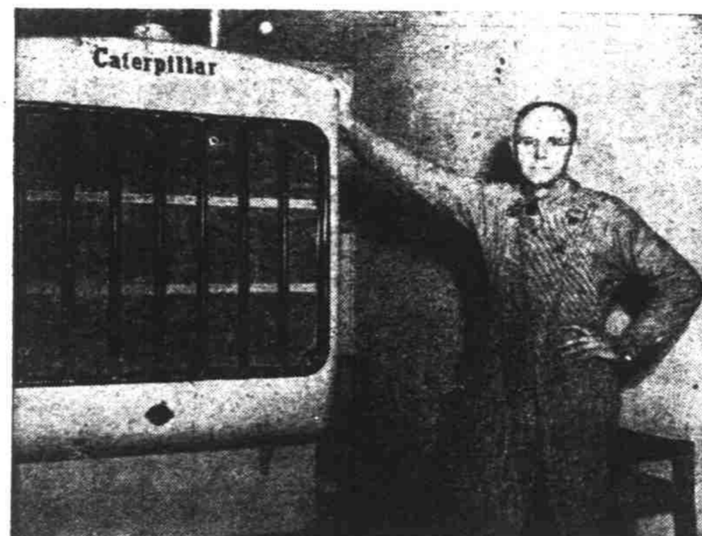
POWER FOR FLOUR and feed. A. D. Gardner shows off new "Caterpillar" D-8800, 102 H. P. engine installed at his mill in Stayton. This engine, replacing ancient water wheel, supplies economical power for entire operation. Picture at right, a view of sacking and tying at the mill.
