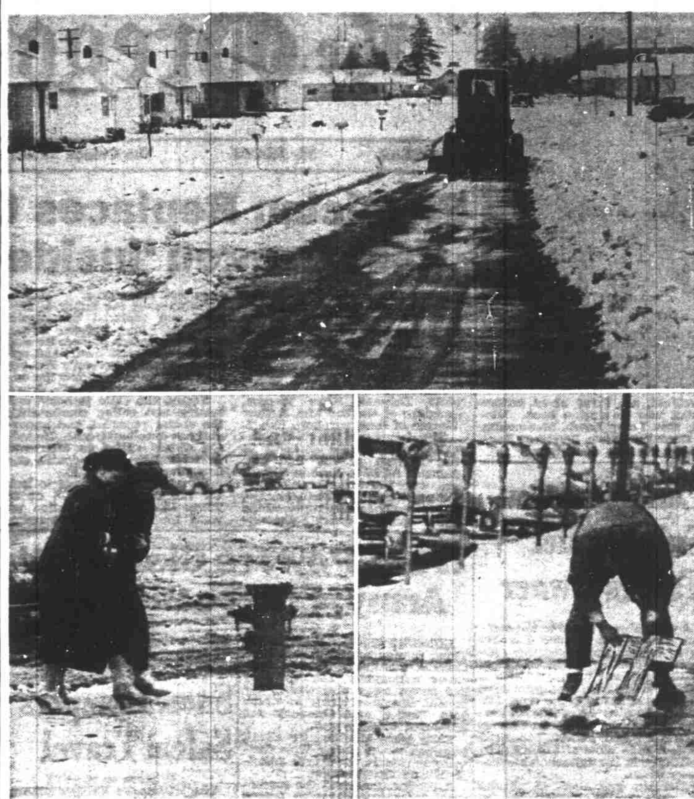
More snow Tuesday saw speedy action by Salem street crews to clear streets in the event the snowfall would be prolonged. In top photo a street grader clears a lane along Tyrone Ave., from N. Front Street to N. Liberty Street. Individually, Salem residents met the snow problem by picking their way gingerly through the slush, above left; and clearing sidewalks with improvised snow shovels, above, right. (Statesman Photos.)
