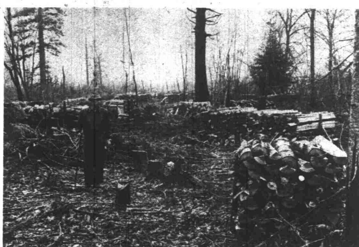
Clair Harvey, wood crew foreman, stands among the hundreds of ricks of cordwood stacked in wood lot 10 miles north of Salem on old North River Road. The wood is being cut for use in the Marion County courthouse by temporarily unemployed men at $7 a cord. About 400 to 500 cords of wood will be cut out of this grove. (Statesman photo).
