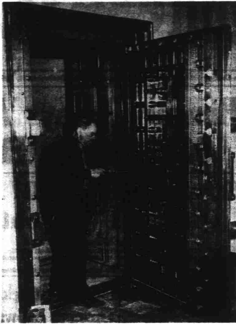
George W. Zerr, master lock and safe smith of Portland, adjusts the huge vault door of the soon-to-open University branch of the Willamette Valley bank at 13th and State streets. Zerr, who has serviced and installed vaults in most Oregon cities, has been a locksmith for 62 years, 34 of them in Oregon. The doors to the new vault weigh about six tons. (Statesman photo.)
