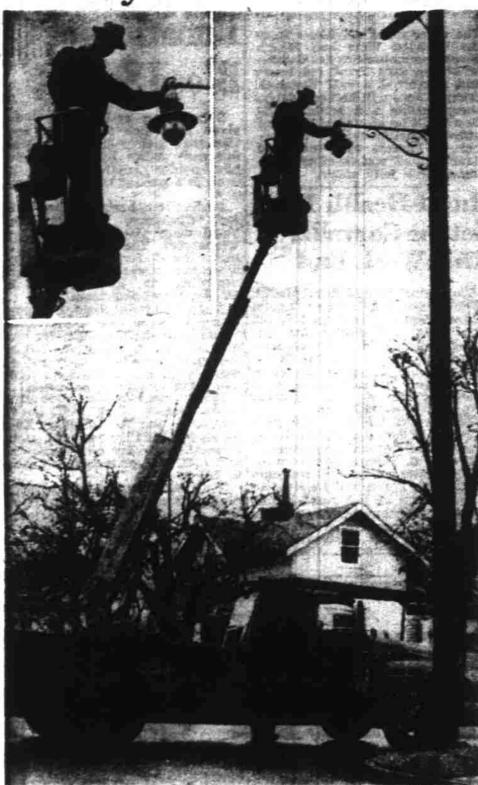
If you have ever wondered how the light globes in street lights are serviced, the answer is above. The hydraulic lift mounted on the Portland General Electric Co. truck can be raised, lowered, tilted and swung about to reach street lights, power lines or tree branches interferring with power lines. Inset shows Eldon E. Hepburn, PGE employe, in the crow's nest. (Statesman photo.)
