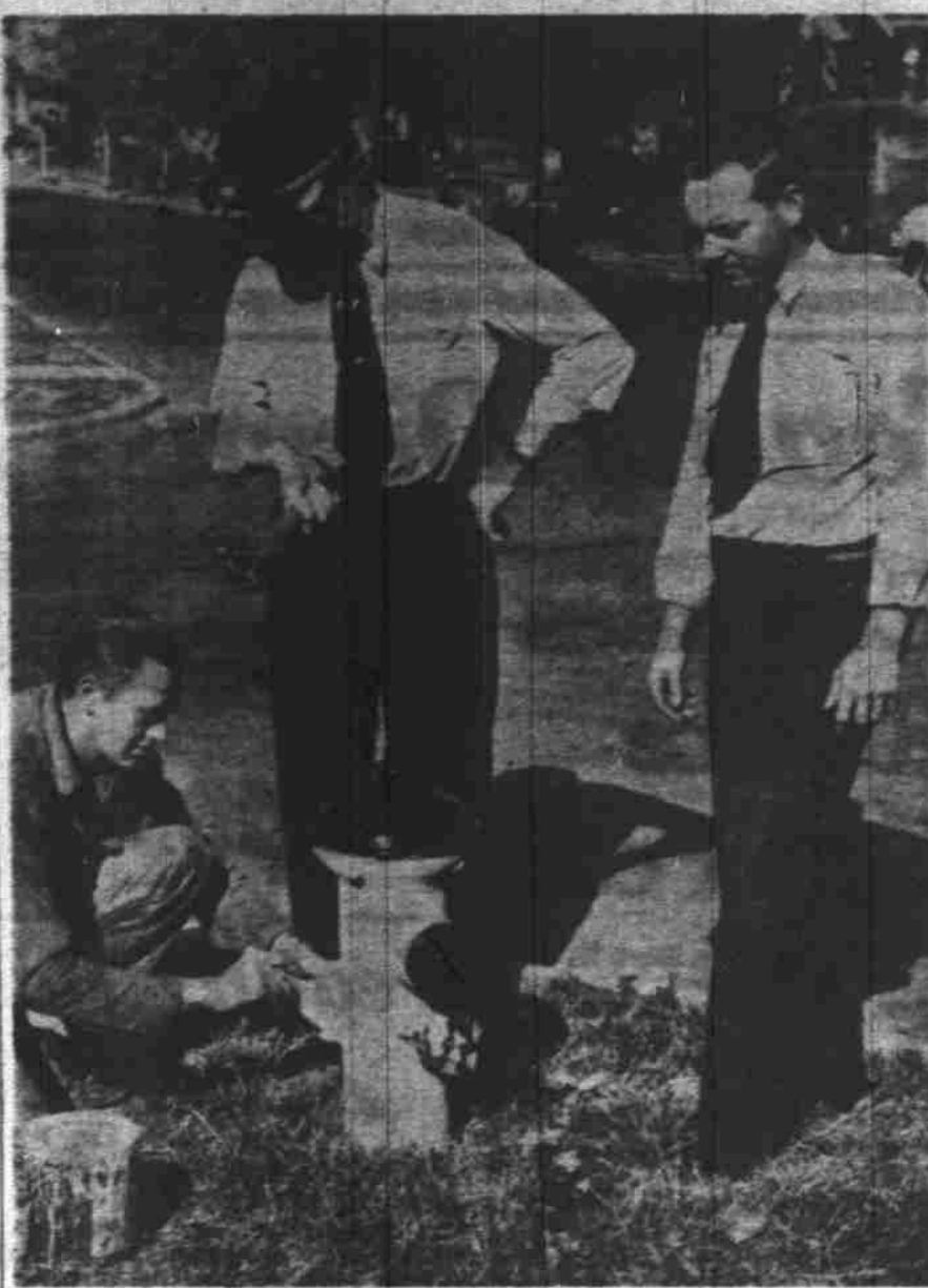
Salem's fireplugs are getting a bright, new coat of yellow reflecting paint so as to loom up at night in a firetruck's headlights. Applying the paint at left is Harold Maynard, 1935 Broadway st.; in center is F. L. Clark, 950 N. 18th st., who is re-threading all the hose connections to prevent any loss of time in coupling hoses to hydrants in an emergency. Also on crew doing work is John Hall, right, 2360 Maple ave. (Statesman photo.)
