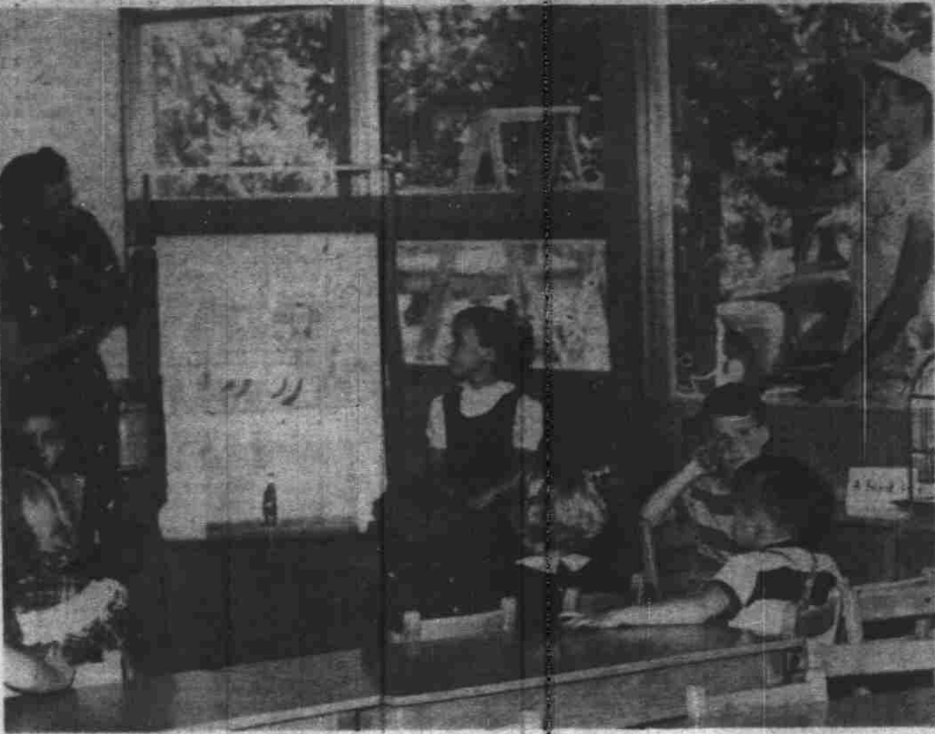
While workmen hurry to finish Baker school, 76 children from the Fairmount district attended their first classes in the new building Monday. Above, a few first graders watch Mrs. Georgia Snodgrass turn a picture scroll as Leo Turner, Salem route 3, paints the trim outside window at right. Although classes are now underway in the latest addition to the Salem school system, much work remains to be done to the building itself. (Statesman photo). (Story on page 2).
