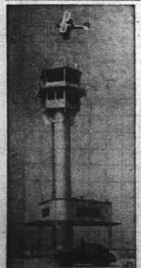
AERIAL PERCH —Control operators will get a bird's eye view of traffic from this new 300-foot-high tower being completed at Sky Harbor Airport, Phoenix, Ariz.
