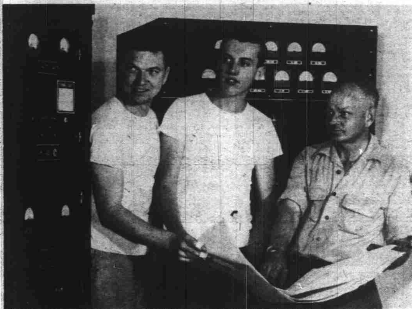
The black cabinets above will house transmitters for a new localizer beam being installed at the Salem airport, and is part of the instrument landing system which, when completed, will allow aircraft to make blind landings. Working on the installation above are, from left, Bob Barnett and John Bowne, both of Oregon City; and Glenn Shoop, Billings, Mont. (Statesman photo.)
