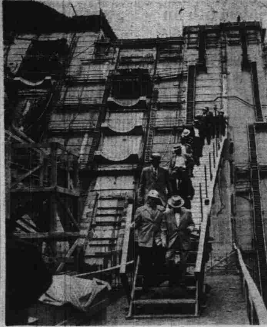
Climbing over the lower face of the new Detroit dam, and peering through the tunnels inside, was a highlight of a four Tuesday sponsored by the Willamette Basin Project committee. Only the men members of the caravan were allowed to go to the "bottom." About a third of the scheduled 1,450,000 cubic yards of cement have been poured. Top photo shows the present stage of construction. (Statesman-Larsen photos).
