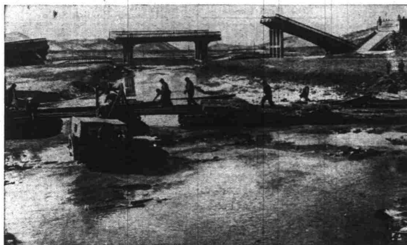
THE ROAD BACK—U. S. Engineers improvise temporary spans bypassing bombed-out bridges.
