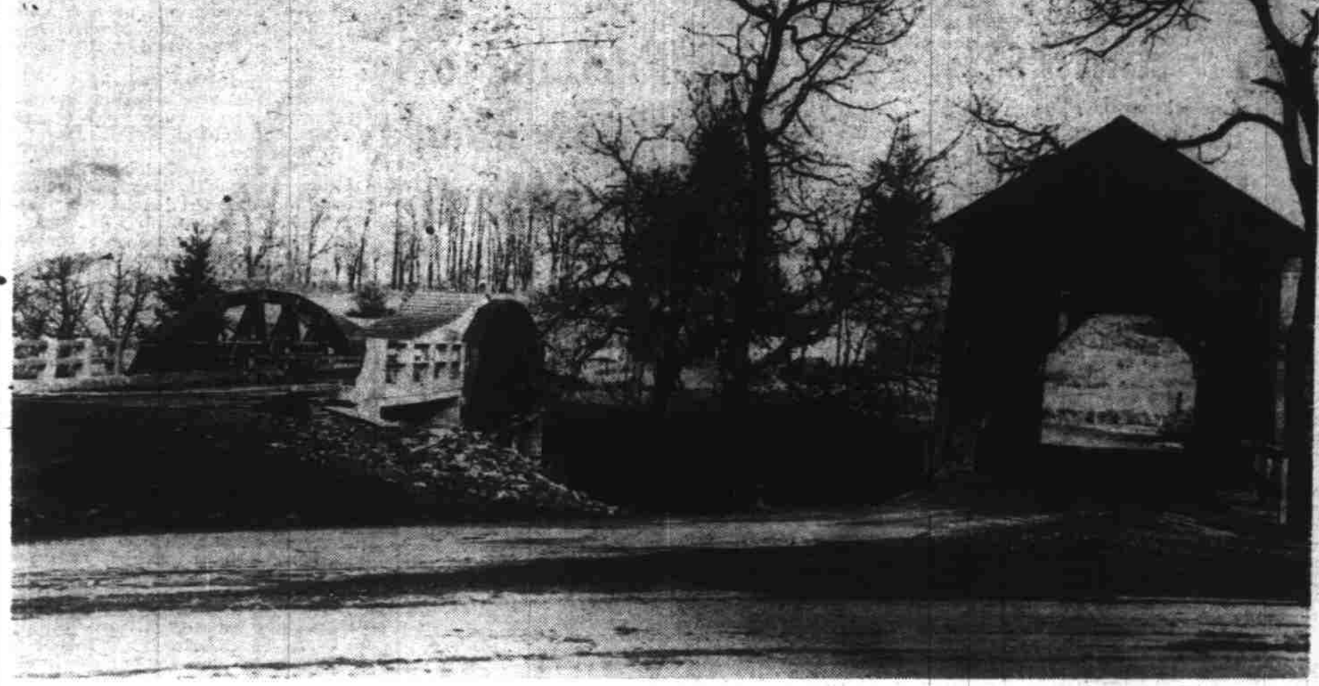
Within a few weeks the new bridge at left will be in use for crossing Butte creek at Scotts Mills, and another of the seldom-seen covered bridges will be gone. This one was built about 1900. The new steel bridge, 90 feet long, was bought from the state and hauled from its original site at Baker. A county bridge crew erected it, put in 40-foot approaches and a concrete deck. Only remaining work is an approach fill to be placed by Clackamas county. The bridge was bought and hauled for about $5,000. Construction brought the cost up to about $25,000 or $5,000 under the original estimate, according to the county court. Pictures of historic spots such as this will play a major part in The Statesman's Centennial editing which will be published on this newspaper's 100th birthday March 25. Extra copies may be reserved now, mailed anywhere in the United States at 15c each. (Statesman Farm Photo.)
