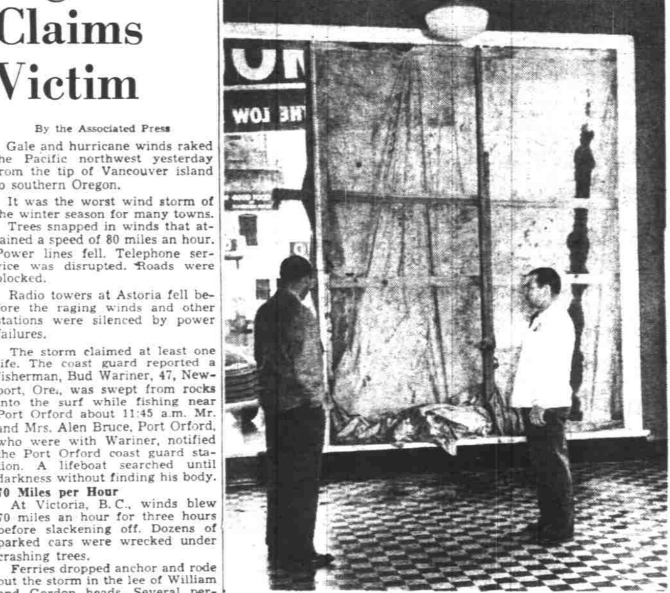
Terrific blasts of wind early Monday morning caused some serious damage as this shattered window at the Stan Baker Motors showroom at Chemeketa and High streets. Surveying the hole left by the 9 by 11 foot plate glass window are Homer C. Stiffler, left, salesman; and Fred Prentice, right, service salesman. The heavy sheet of glass narrowly missed a new car sitting on the showroom floor. (Statesman photo.)
