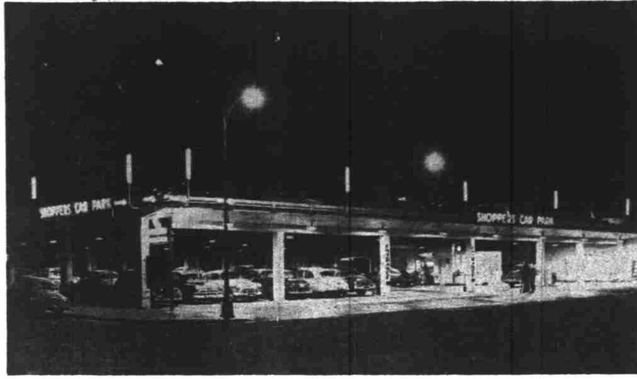
This new 250-space Shoppers Car park was dedicated to Salem shoppers with appropriate ceremony Saturday. A large crowd passed through the double-decked structure occupying a quarter block on the southwest corner of South High and Ferry streets. Favors were given out and city officials participated in the dedication program arranged by Thomas A. Roberts, manager.
